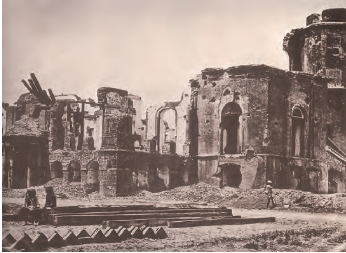
Fig. 17 – Ruins of the Residency in Lucknow
